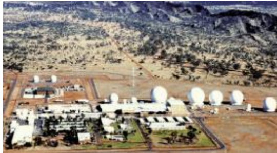
Pine Gap, central Australia
